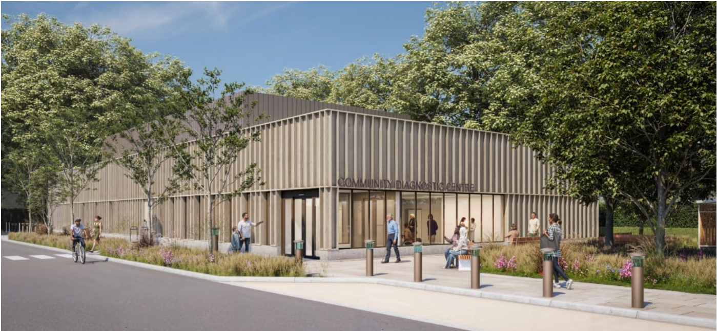
Corby Community Diagnostics Centre - Modular build
